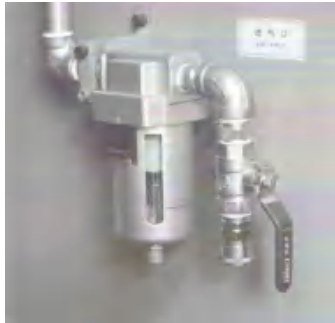
Air filter, used to filter moisture from the air, discharged once a day
